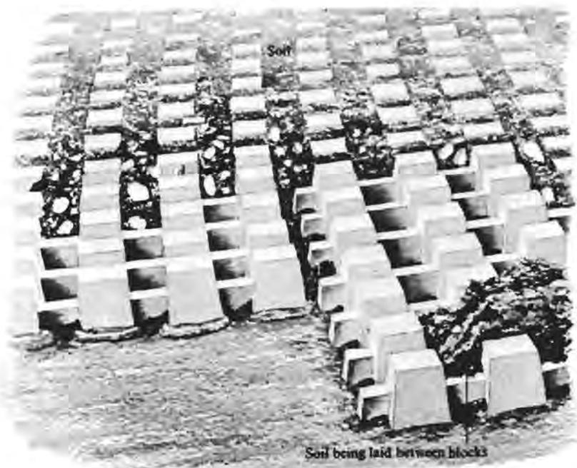
Figure 4. Porous pavement (Source: Dunne and Leopold, *Water in Environmental Planning*, Copyright W.H. Freeman Co., 1978).
